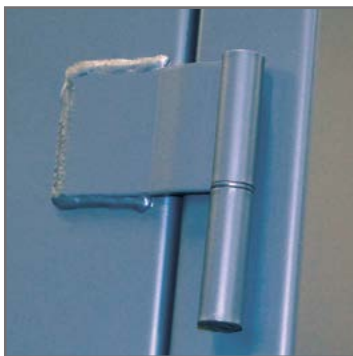
Welded on hinges
